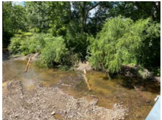
Single log vane deflectors installed at the Woodcock Creek site.
