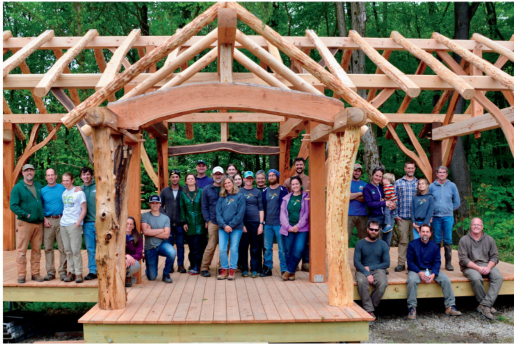
Volunteers enjoy their accomplishment and comradery after working shoulder-to-shoulder to raise TLC's new outdoor classroom. Photo by Leo Glenn.
